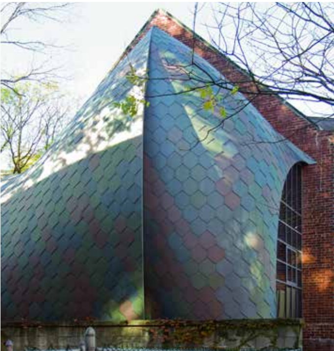
Extension of an architectural office, Hoboken - USA
